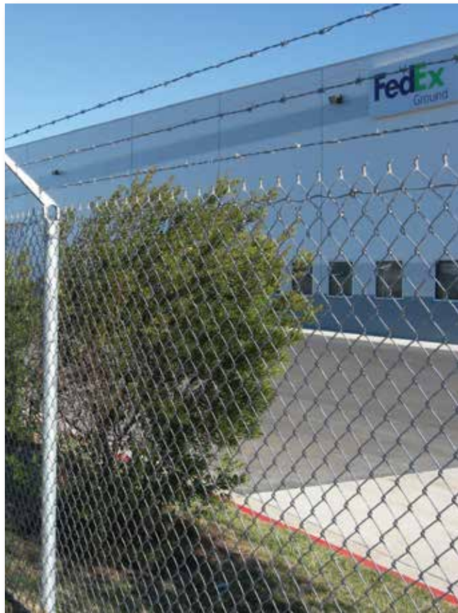
FEDEX FACILITY - AUSTIN, TX
